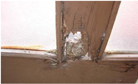
Termite and weather damaged windows
